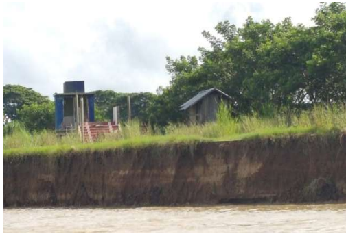
Plate 3: allocation the Monastery by Bank erosion at Kyaukye Village (27.6.17)
